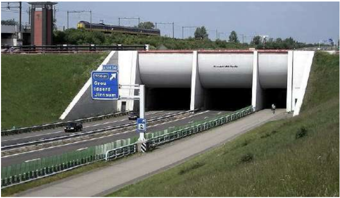
Aquaduct Mid-Fryslan, Grou
