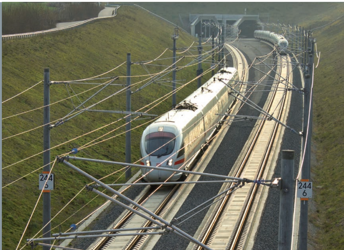
New line Erfurt-Leipzig/Halle (VDE8.2): two ICE trains run in parallel for the route opening on 9 December 2015 Title: Froschgrundsee Viaduct, new line Ebensfeld-Erfurt (VDE 8.1) 2016
