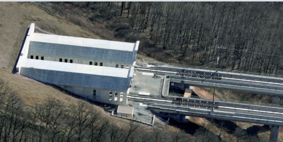
Hood structures as noise protection measure and extinguishing system, Bibra Tunnel 2012/2014
