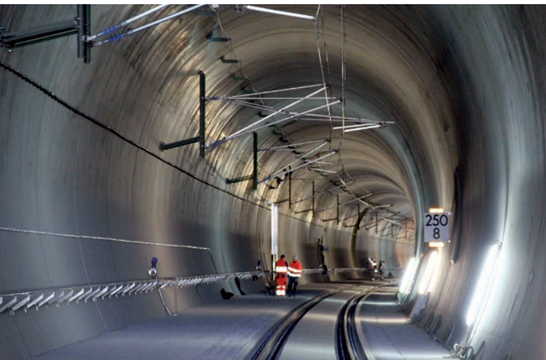
Tunnel that can be used by road vehicles, Osterberg Tunnel 2014, new line Erfurt–Leipzig/Halle (VDE 8.2)
