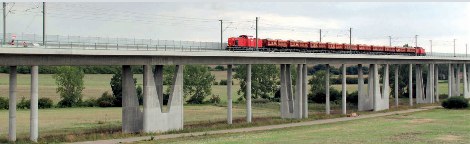
Gänsebachtal Railway Bridge during a load test run, new line Erfurt–Leipzig/Halle (VDE 8.2) 2014
