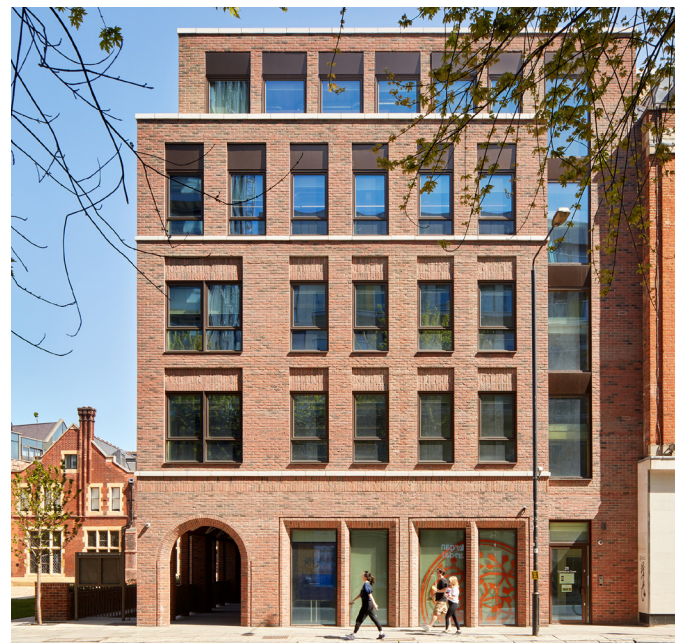
28 Commercial Street, Whitechapel, Tower Hamlets (Platform 5 Architects)
